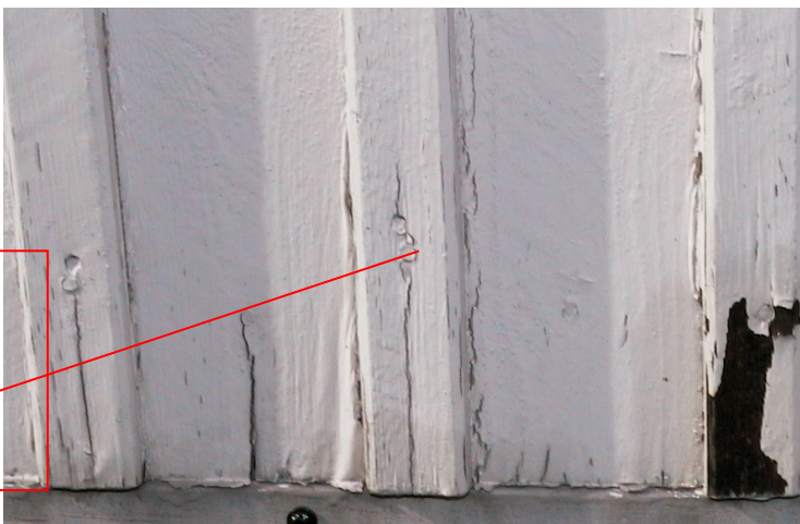
Picture 1. Paint that is degenerated.
